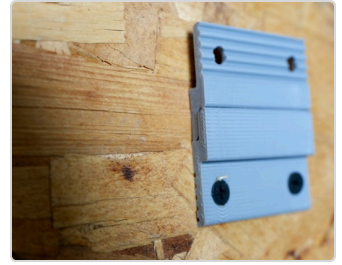
Wall clip screwed in, stepped edge facing up
